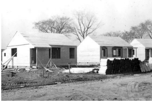
Figure 1- Construction of Victory Houses On Normandy Boulevard in 1947.
